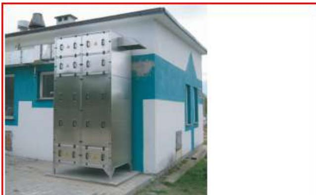
Figure 4: Full scale photo ionisation plant for headworks building in Poland
