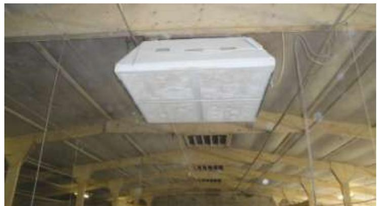
To reduce the effect on the local inhabitants a photocatalytic reactor removes the odours, ammonia and the health hazard of fungal spores. Test rigs have been trialled with results giving 80% odour and ammonia reductions whilst filtering out spores.
